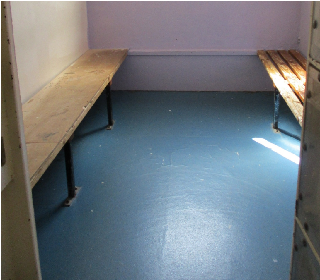
Seating in health care waiting room
