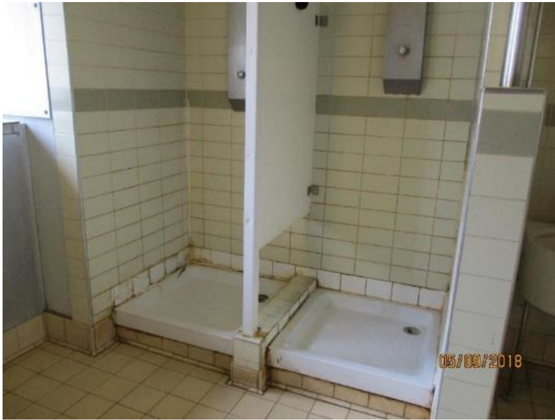
D wing shower room – 2018
