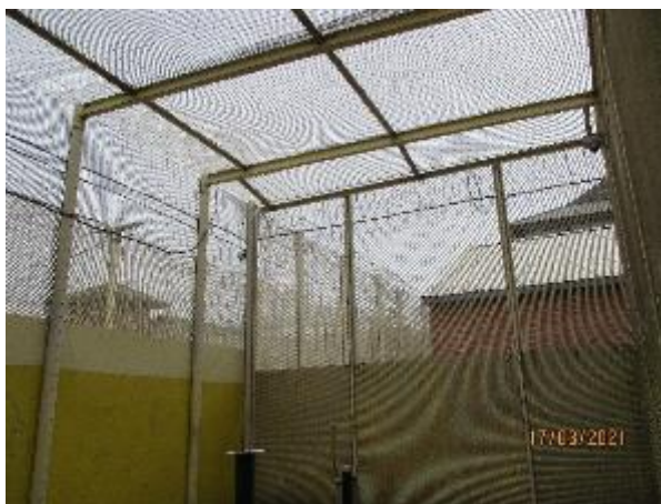
Segregation unit exercise yard
