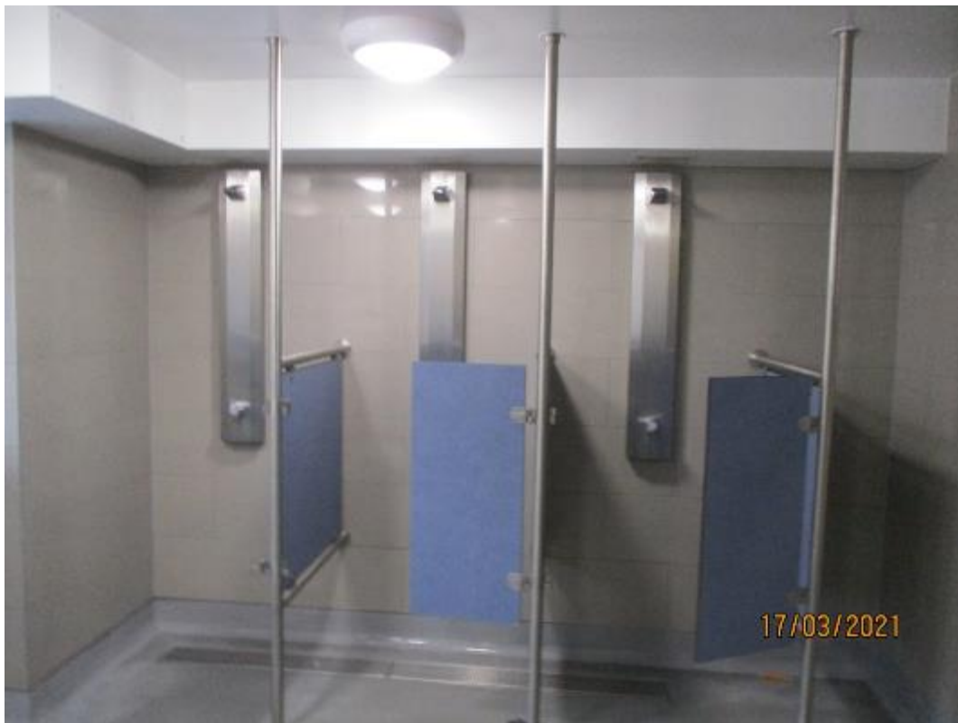
D wing shower room – 2021
