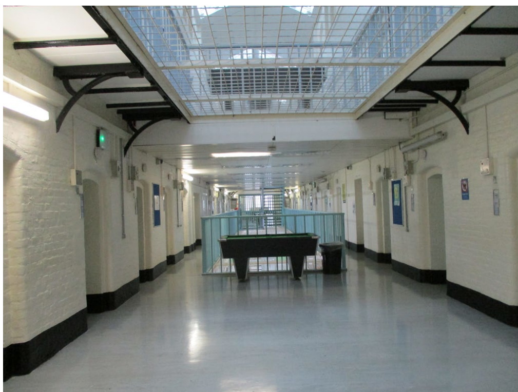
B wing upper landing
