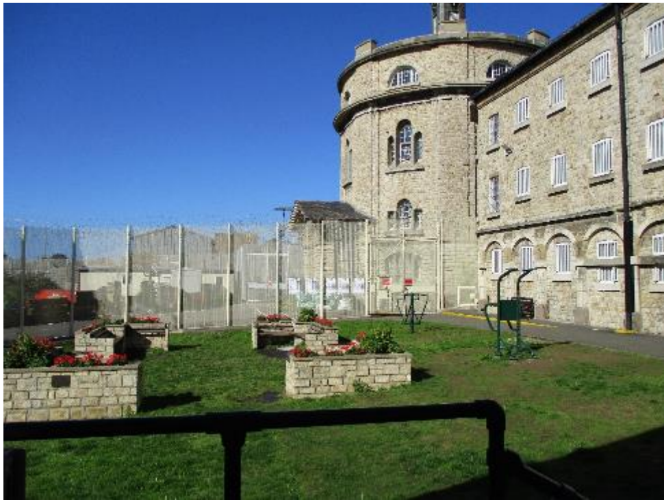
Weald House exercise yard
