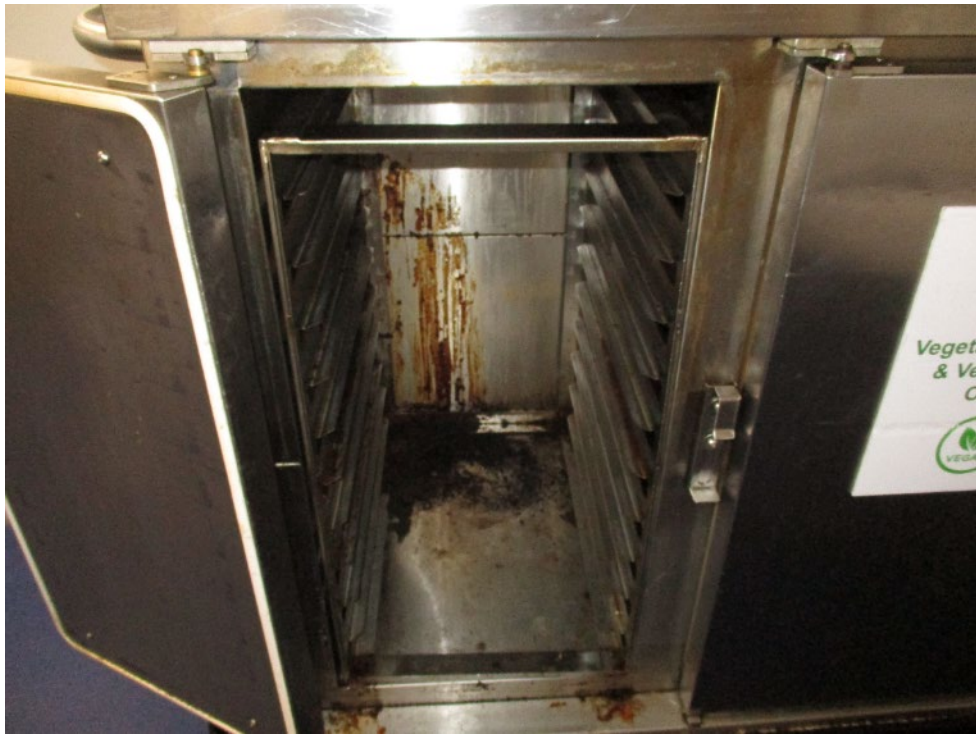
Dirty trolley in kitchen
